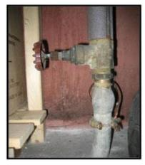
Lead service lines can be connected to the residential plumbing using solder and have a characteristic solder "bulb" at the end, a compression fitting, or other connector made of galvanized iron or brass/bronze.
