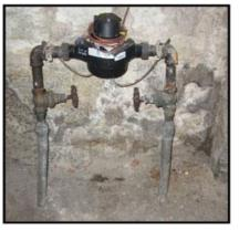
Lead service lines often end just inside the front or side wall of the home, but may extend further into the building as shown, where the lead service line comes out of the basement floor to the water meter and then back into the floor, continuing further into the building.
