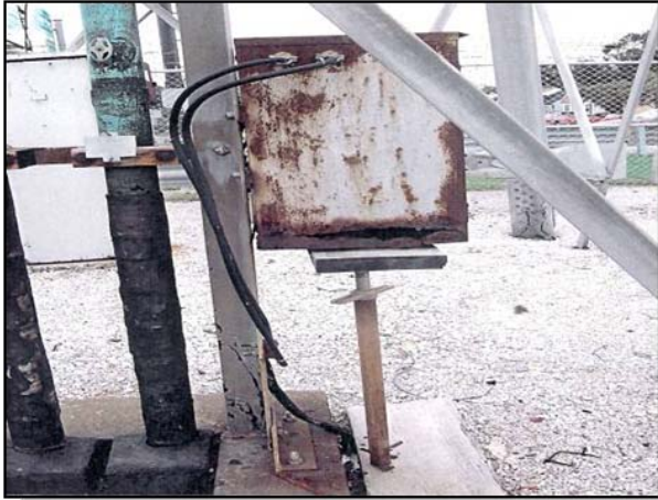
Rusted cathodic protection device insecurely mounted on a jack stand
