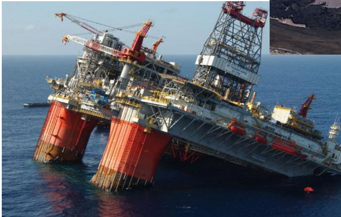
BP's Thunderhorse platform listing in Gulf of Mexico after Hurricane Katrina
