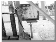
Rusted cathodic protection device insecurely mounted on a jack stand
